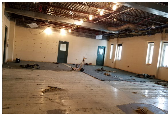
Hall Tech room 222 is under construction.
