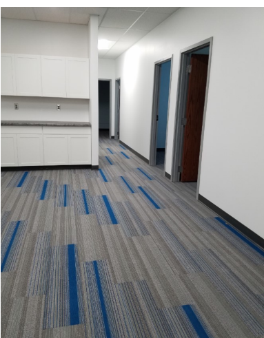
Whitaker 125 is almost done!
