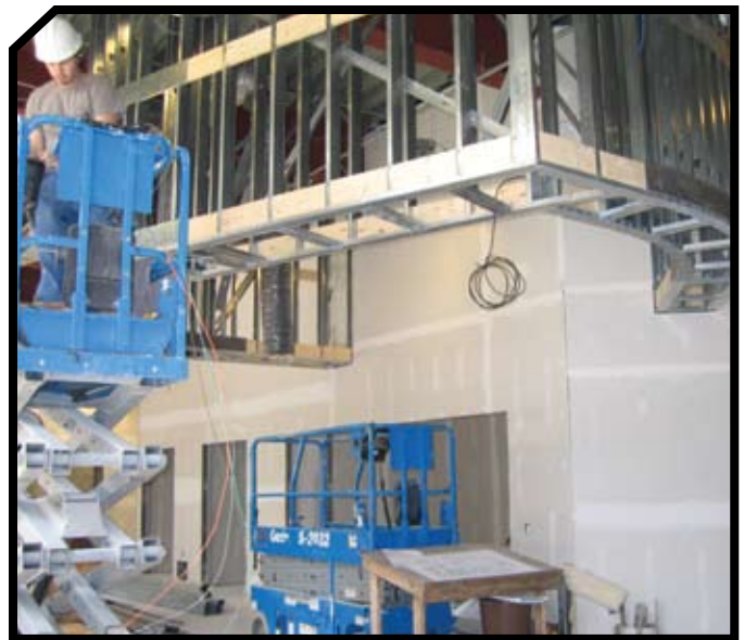
The walls and overhead structure are going up on the welcome center site.
