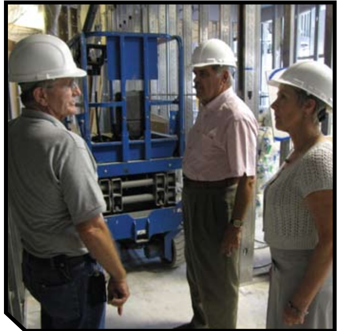
Denis Deslongchamp, campus director of facilities management, left, gives a tour of the renovations work to Dr. Frank J. Dixon, long-time HACC benefactor, center, and college President Edna V. Baehre, Ph.D.
