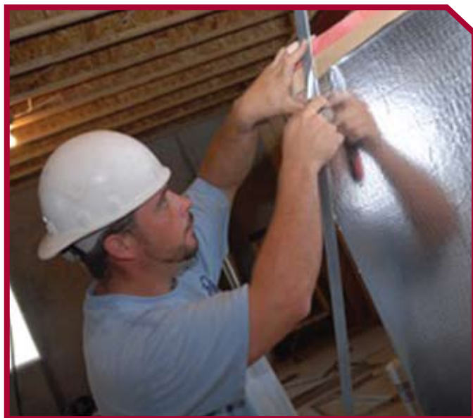
Dan Ball installs ducts for air conditioning at a construction site in York.
