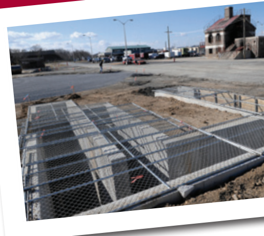
The trench rescue laboratory will include above-ground and under-ground trenches and manholes, pipes and simulation props to replicate disaster scenarios.
