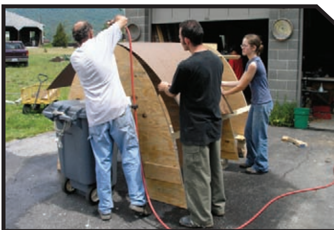
Jim Lard, left, gets assistance from student volunteers in building a wooden frame for the shape of the kiln, which is built of firebrick (top right). The frame was removed after the kiln was constructed.
