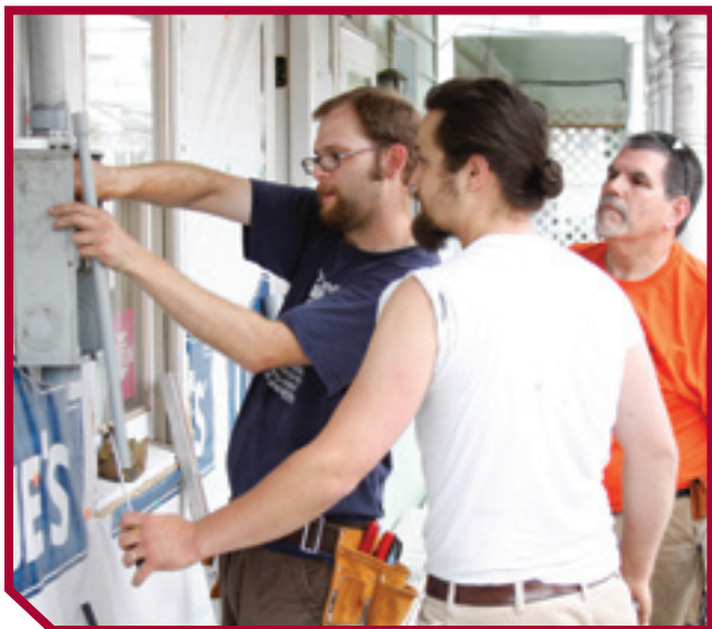
Students in Rob Meyers' residential electrical wiring class work on wiring a Habitat for Humanity home on Zarker Street in Harrisburg.
